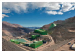
Caserones Copper Mine
