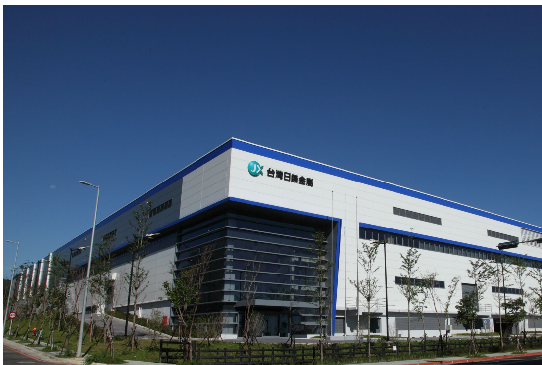
Exterior view of Nikko Metals Taiwan
