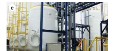
Rinse Recycling System (e) —to reduce industrial water consumption
