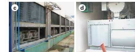
Upgrade from an old chiller (c) to a more efficient turbo-chiller (d) for lower electricity usage
