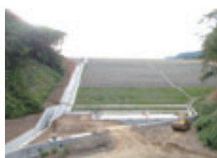
Restoration project of the impoundment (July 2013)
