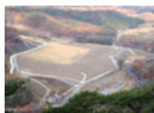
The impoundment after completion of the project (November 2012)
