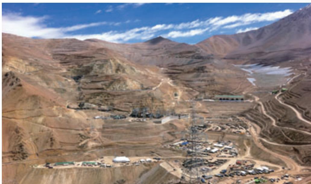
Panoramic view of the Caserones Copper and Molybdenum Deposit (in March 2013)
