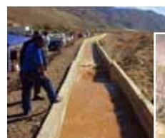
Irrigation channel repaired with reinforced concrete
