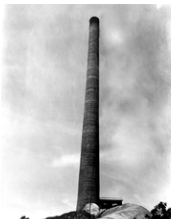
The Giant Stack of Seki, which adopted the same steel-reinforced concrete construction as the Hitachi stack
