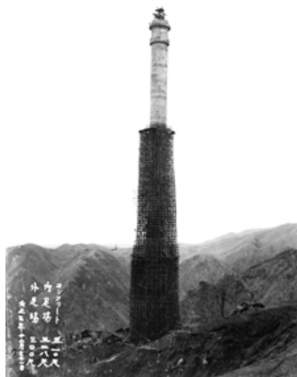
The Hitachi Giant Stack, unusual at the time for its steel-reinforced concrete construction
