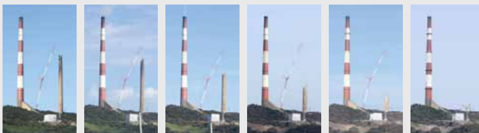
Dismantling the First Giant Stack
