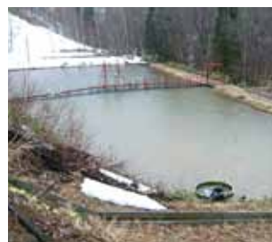
Settling pond for solid-liquid separation of neutralized water
