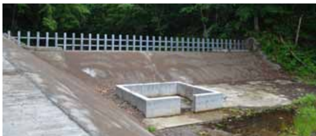
Hanawa Mine, Tanosawa Tailings Dam, where torrential rain countermeasures were implemented (top) Embankment and emergency drain (bottom) Trash rack to stop flow of tree debris in torrential rain
