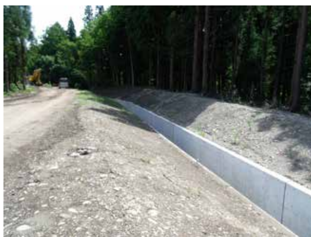
Completed drain as torrential rain countermeasure at Tashiro Mine
