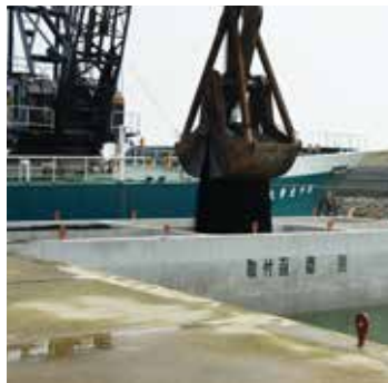
Filling a caisson with slag
