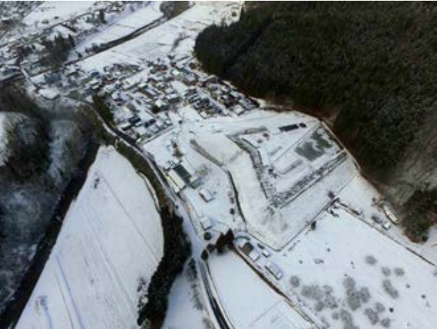
Earthquake countermeasures at Namariyama Mine, Oyu 1st and 2nd Tailings Dams
