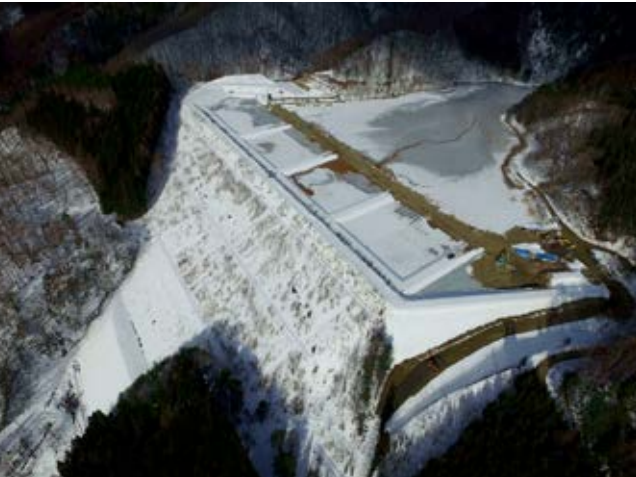
Earthquake countermeasures at Hanawa Mine, Nakanosawa Tailings Dam
