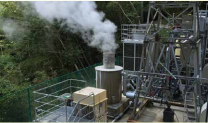
Binary cycle power generation system using heat from Shimoda Hot Springs
