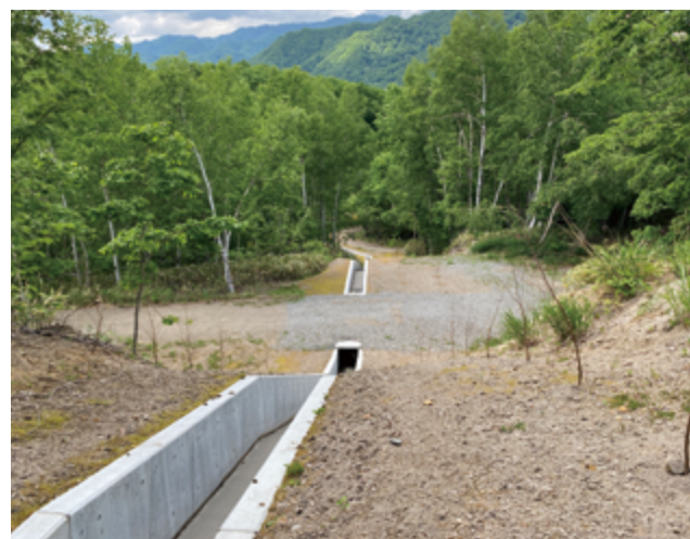
The drainage canal of the Toyoha Mine Ishiyama tailings dam, completed in FY2022
