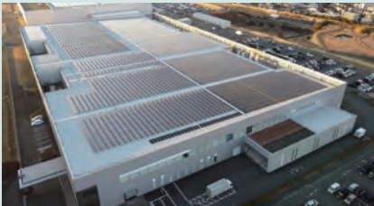
Solar power generation equipment installed on the roof of the Kakegawa Works
