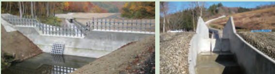
Countermeasure construction: Installation of check dams (driftwood stopper) Countermeasure construction: Upgrading drainage channels
