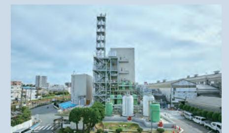
New catalyst production facility at the Chigasaki Plant (Kanagawa Prefecture)
