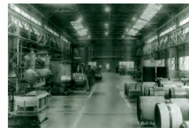
Kurami Works just after completion
