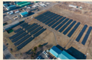
Solar power generation system installed by a PPA operator
