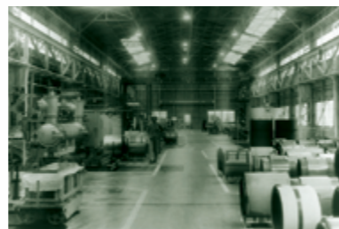
Kurami Works just after completion
