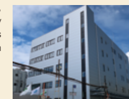
Analysis center building
