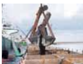
Filling a caisson with copper slag
